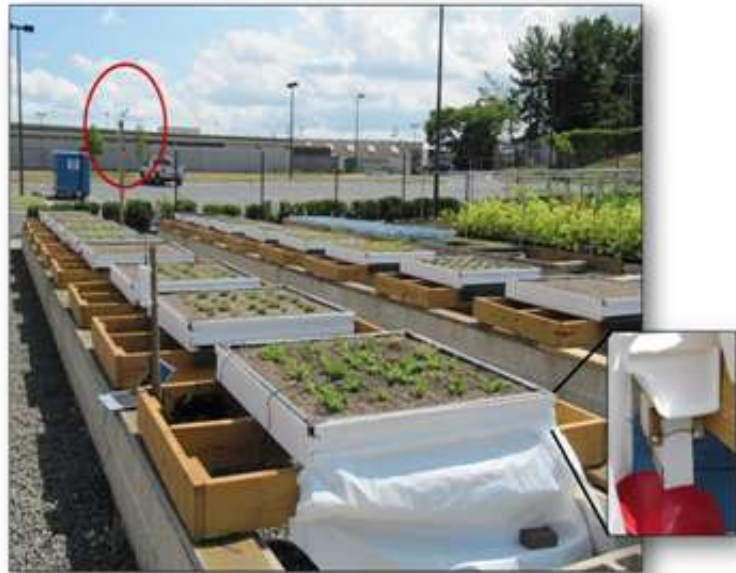
Figure 3. University of Maryland Green roof experimental site. Insert shows rain gauge installation on the gutter to collect stormwater runoff. Each replicate platform collects substrate moisture and temperature data from four Echo-TM sensors, with a substrate-specific calibration.
